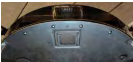
Example of top repair
