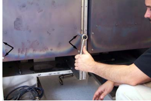
Removing bolts (arrows) securing flue to frypot.
