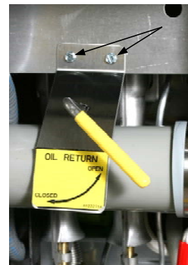
Oil-return handle bracket and screws.
