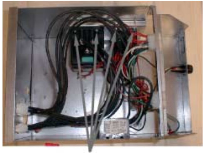
Contactor mounting screws
