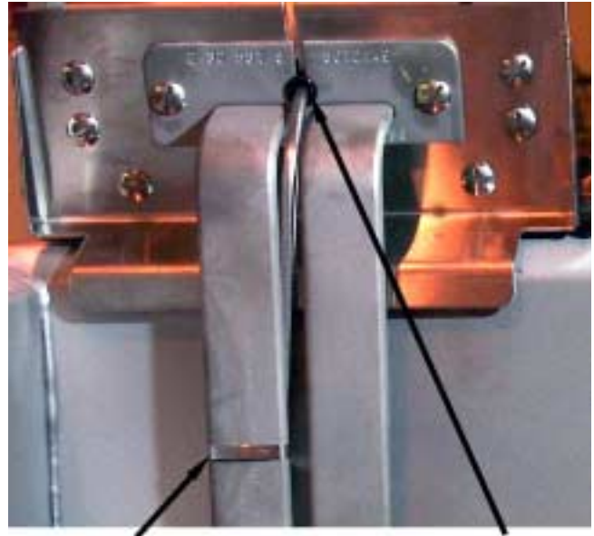
Secure probe to element with metal Ty-Wrap
