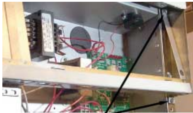
Screws securing control panel frame
