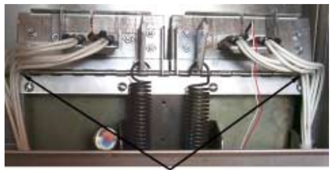
Proper element-wire routing is essential to prevent wire chafing while raising and lowering elements.
