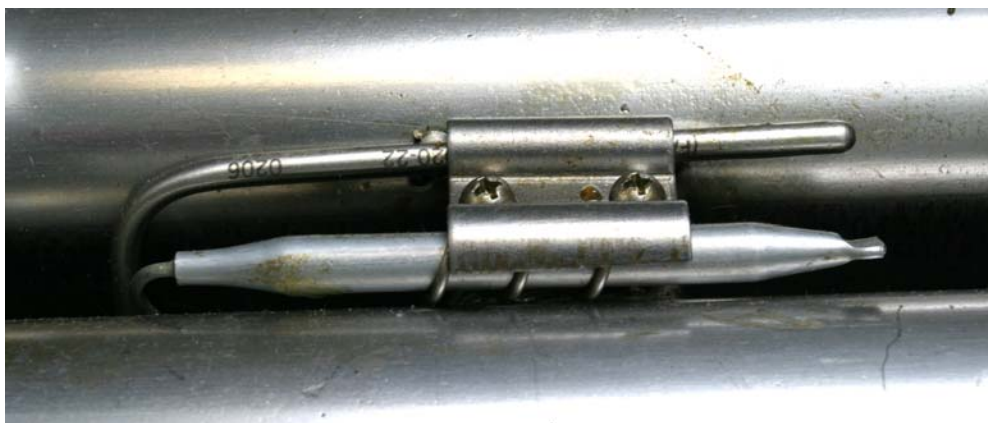
Typical high-limit/sensor probe locations and mounting hardware.
