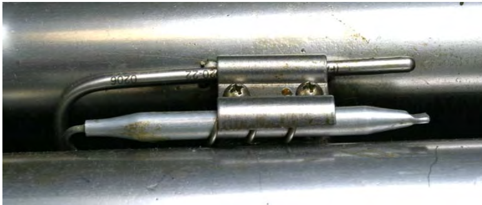
Typical high-limit/sensor probe locations and mounting hardware.
