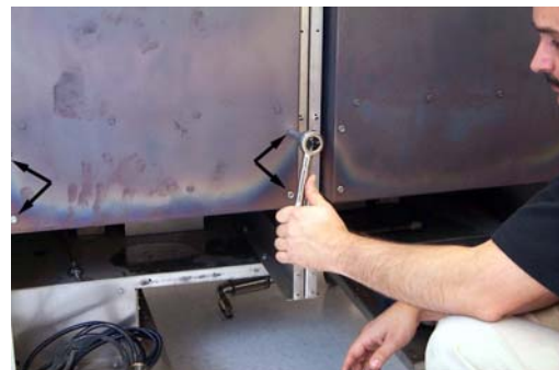
Removing bolts (arrows) securing flue to frypot.
