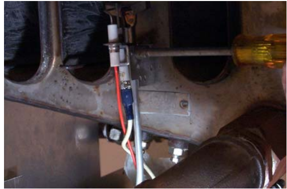
Removing electronic/standing pilot assembly.
