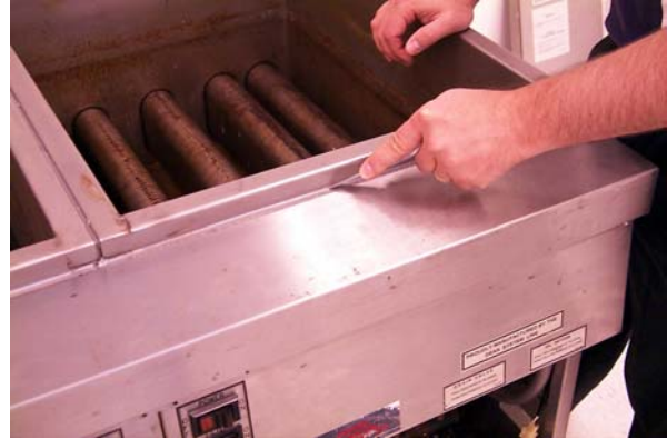
Cutting frypot seal prior to frypot removal.
