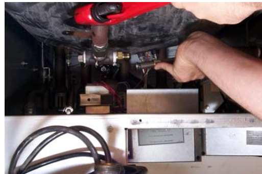
Turn the oil-return valve slightly outward to facilitate removal of the oil-return line.
