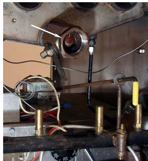
Ball retainer nut (arrow) on drain valve.
