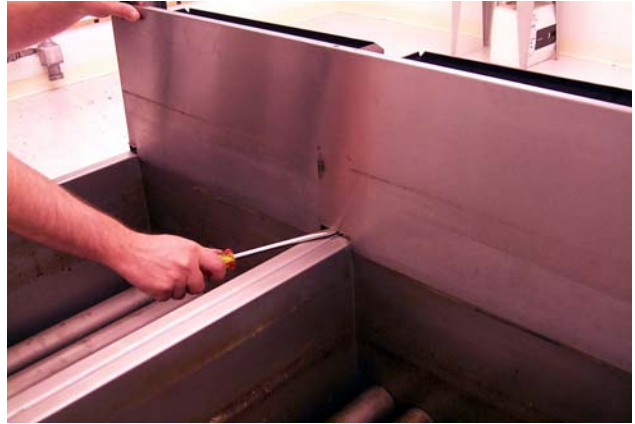
Removing flue cap.
