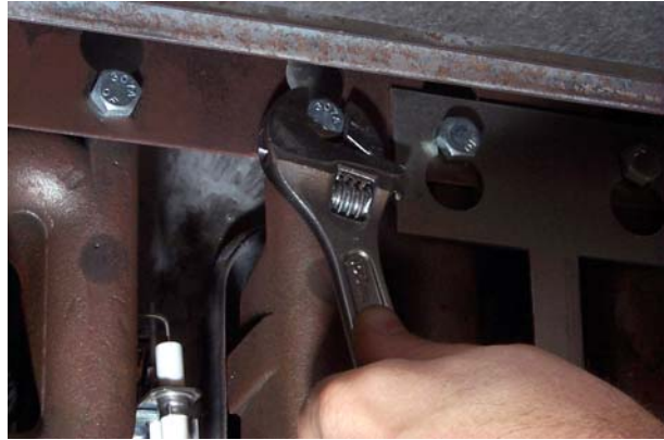
Loosening burner bolts prior to burner removal.
