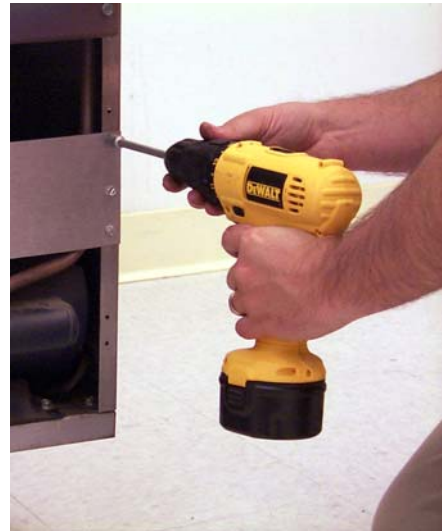
Removing gas manifold shield.
