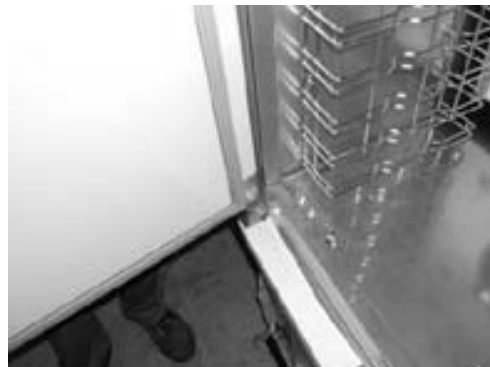
9. Install the door, inserting the top hinge into the prepunched holes, aligning the left lower hinge with the prepunched holes.
