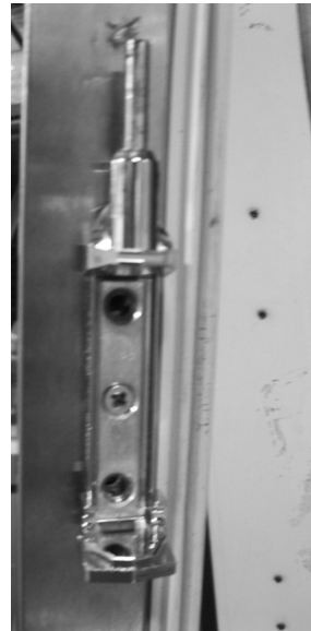
Photo 2. Rotate hinge 180°
