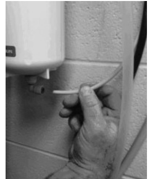
Insert reject line into elbow. Flow control installation is now complete.
