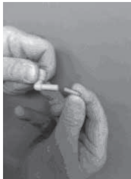
Insert Flow Control Into Elbow
