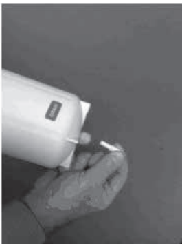
Remove RO Membrane Cartridge Drain Plug
