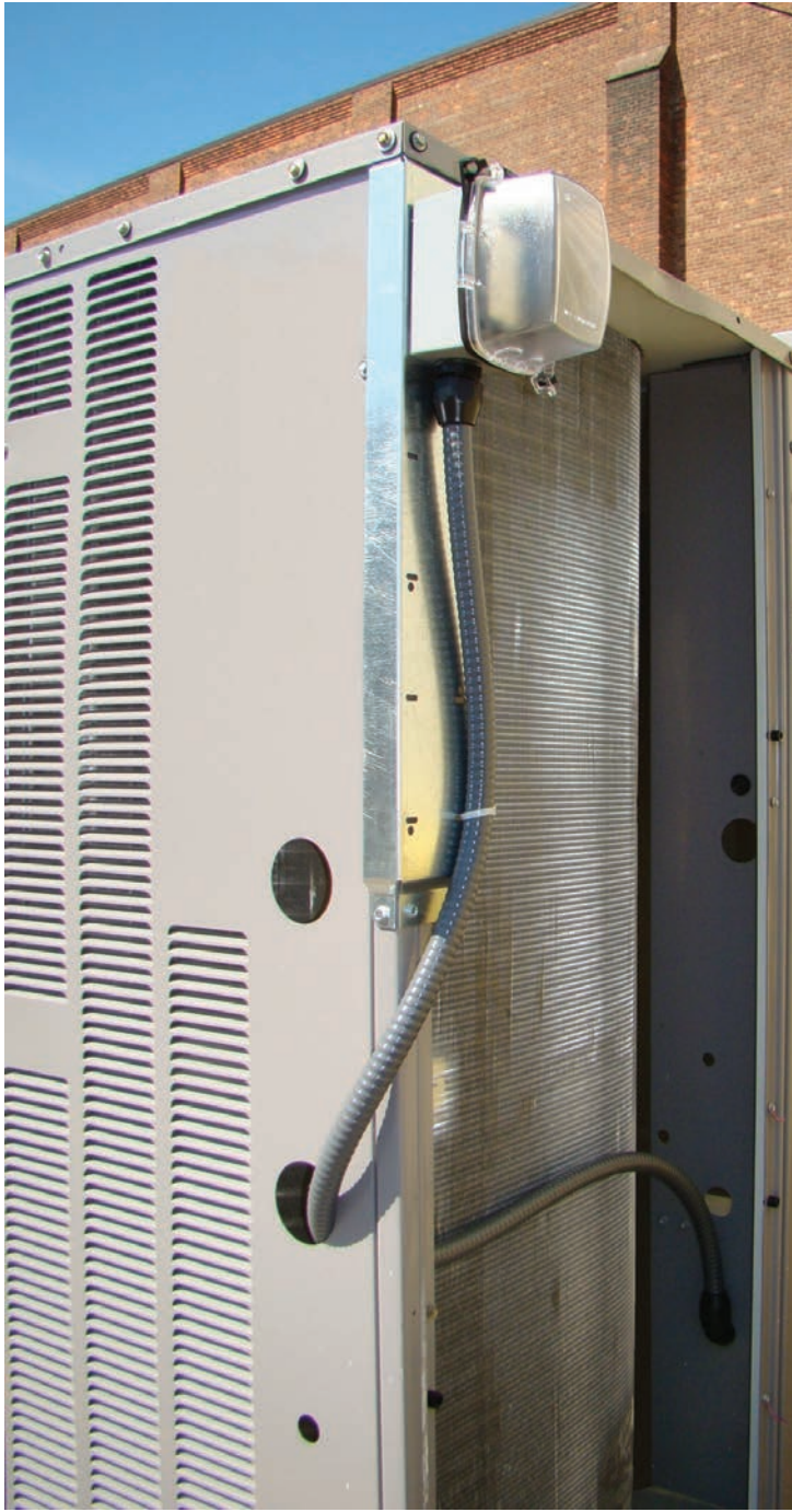
Fig. 5 - Accessory Kit Mounted under Top Cover Flange on Large Chassis Unit (Liquid tight conduit and connector field supplied)
