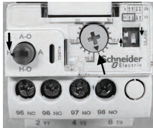
Fig. 33 — 042-1 Units (Size 042, 208/230V) Overload Settings
