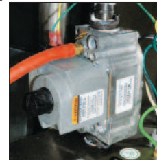
7. Gas Valve (showing hose for pressure tap)
