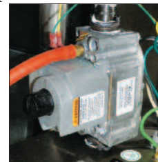
7. Gas Valve (showing hose for pressure tap)
