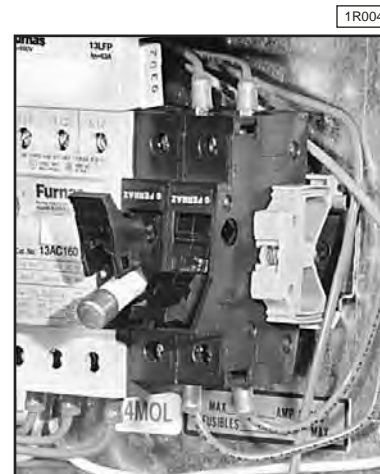
Figure 1 Fuse Blocks
