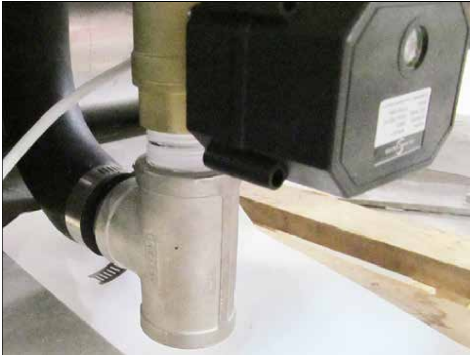
Fig. 7 - 1" NPT electric drain valve connection
