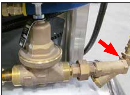
Fig. 8 - Standard and Heat Recovery hot water connection
