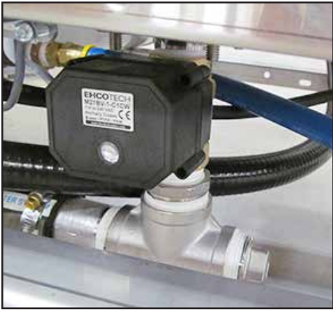
Fig.15 - Single tank drain connection
