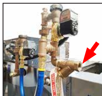
Fig. 9 - Hot water connection no internal booster
