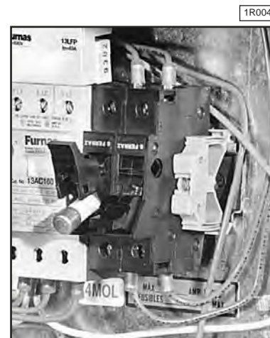
Figure 1 Fuse Blocks
