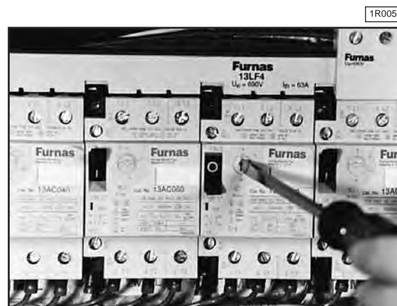
Figure 2 Motor Overload
