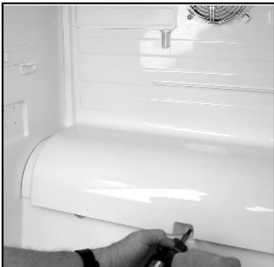
4. Remove the single screw securing the evaporator cover.
