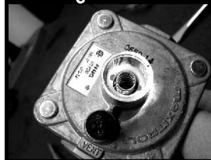
8. To adjust pressure: Remove brass cap & turn white plastic part inside the stem of regulator
