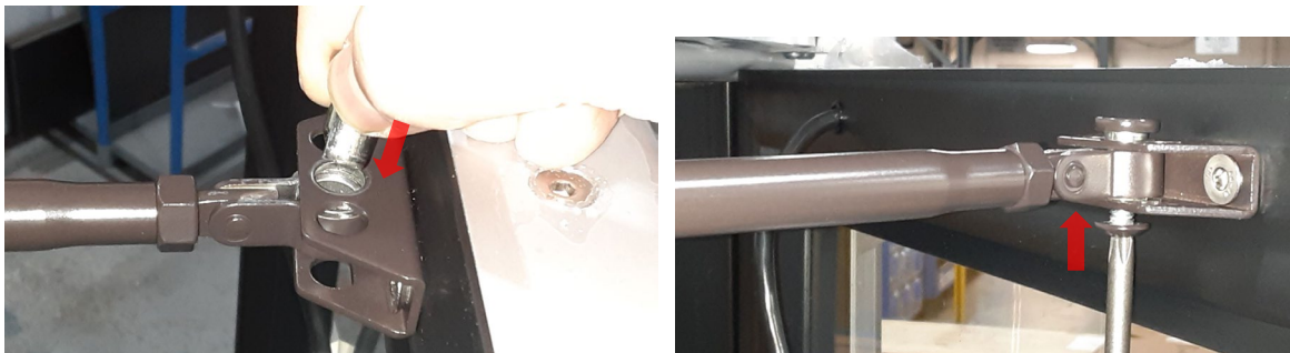
Figure 5.5: Installing Door Closer Arm to Door Bracket
