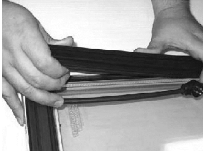
Figure J.4 – Installing replacement Plastic Cover
