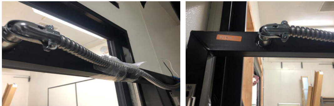
Figure 2.10: Conduit Exit location
