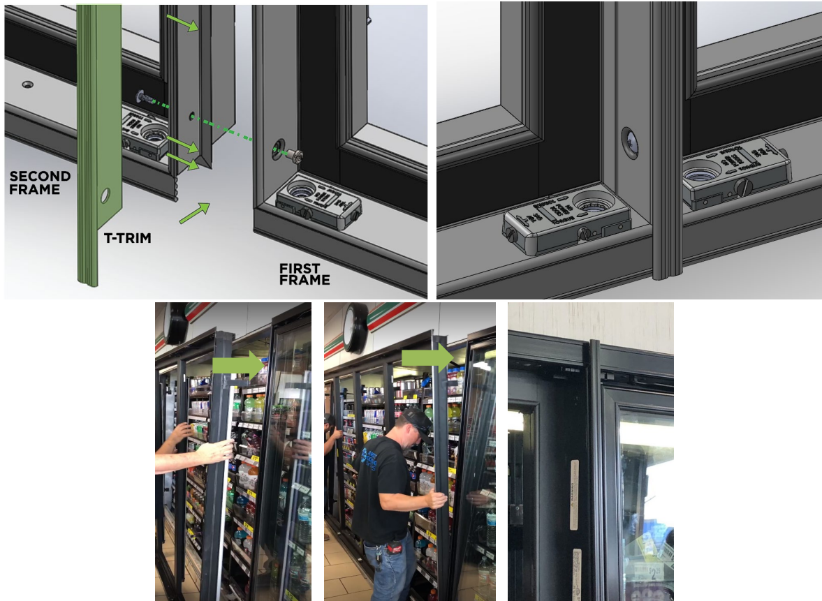
Figure 2.6: T-Trim installation
