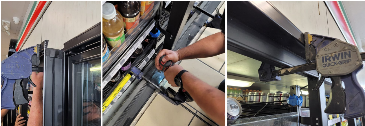
Figure 2.2: Clamps to insert Frame into Net Opening
