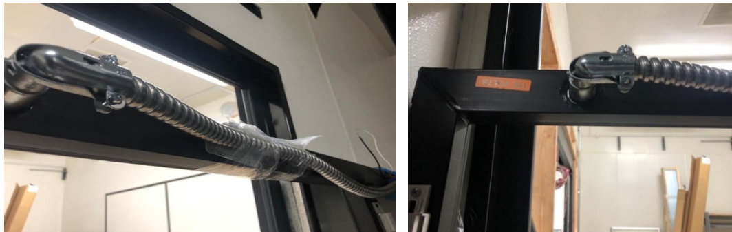
Figure 2.11: Conduit Exit location
