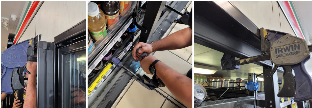
Figure 2.2: Clamps to insert Frame into Net Opening
