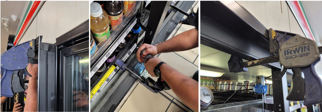
Figure 2.2: Clamps to insert Frame into Net Opening
