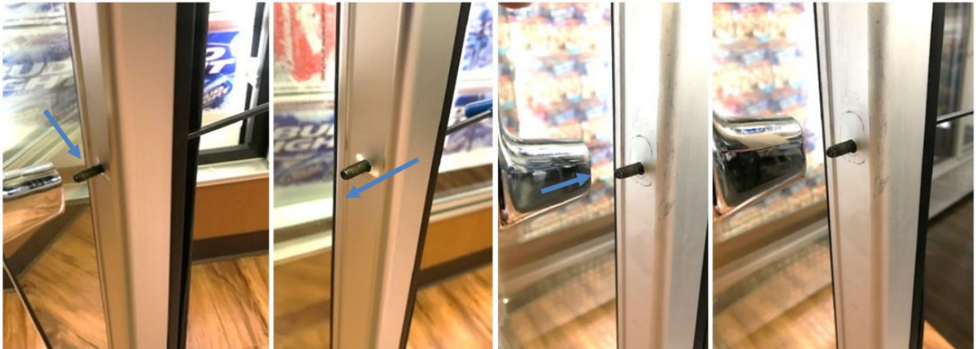
Figure F.2 – Expose screws and secure the new handle
