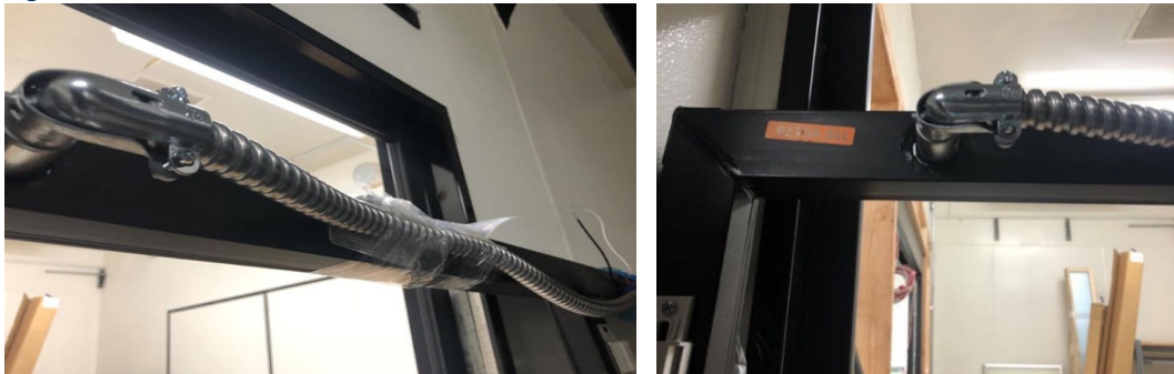
Figure 2.10: Conduit Exit location
