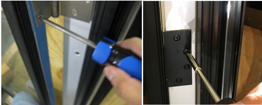
Figure 18.13: Mounting Door Hinges to Frame
