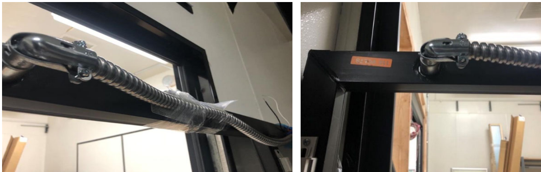
Figure 2.10: Conduit Exit location
