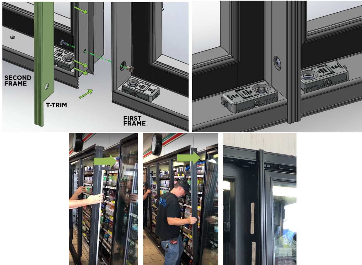
Figure 2.6: T-Trim installation
