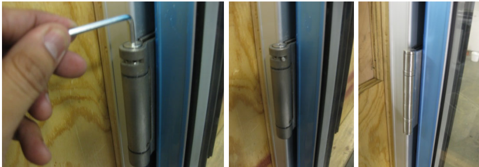
Figure 18.16: Torquing Hinges
