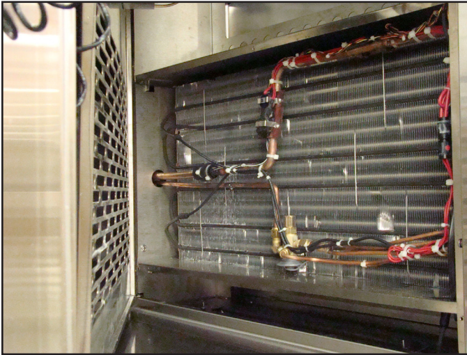
Evaporator Coil
