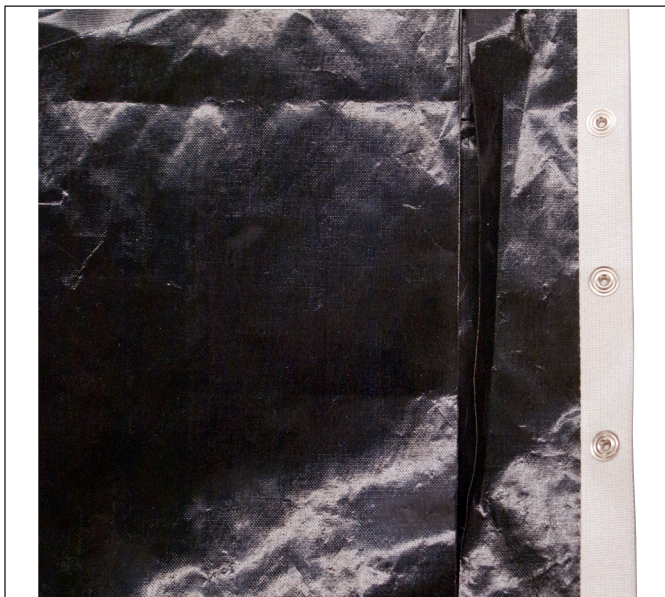
BELT IS TORN AND FOLDED. REPLACE BELT.
