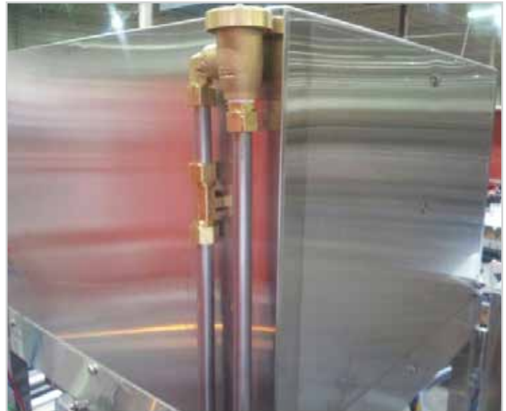
ASSE approved vacuum breaker (backflow preventer)
